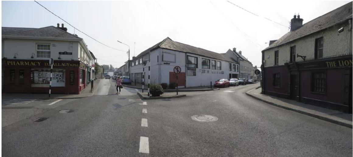
Fig 25: View of New Lane and Bridge Street showing vacant buildings and narrow footpaths and a lack of planting.
